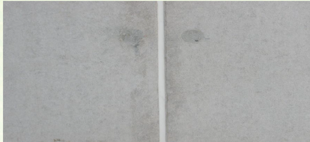
Apparent sealed joints
